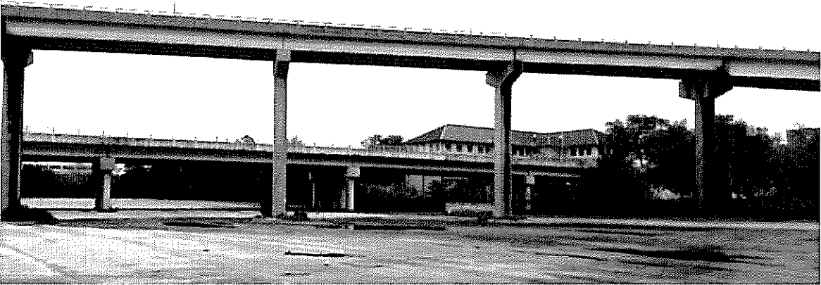
Internal picture of the subject site facing northeast
